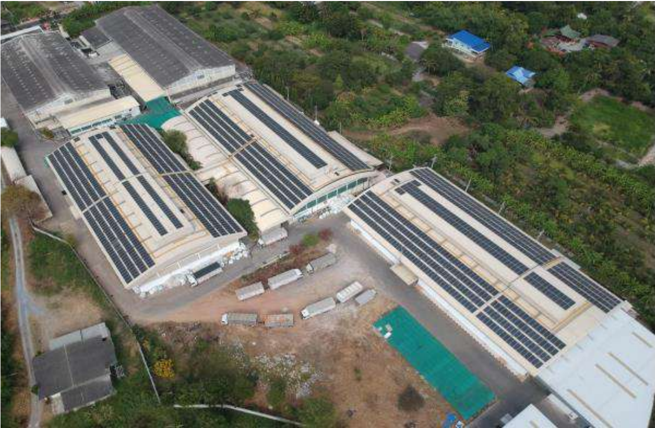
Installation of solar panels on the roof of the company's production building 3 buildings
