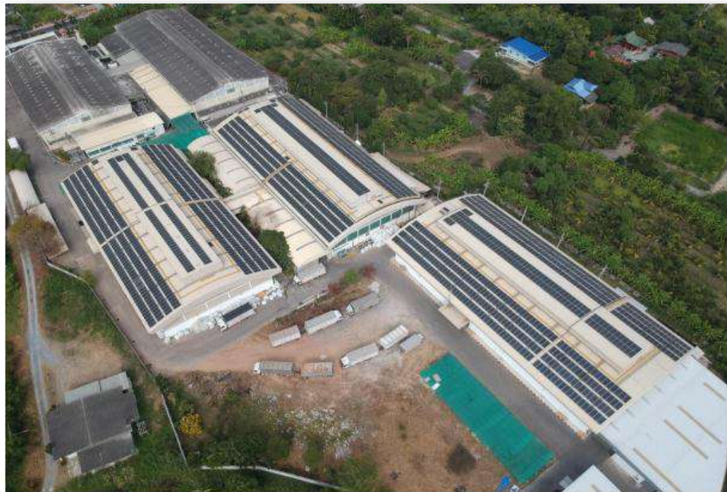
Installing the company's solar panels on Building
